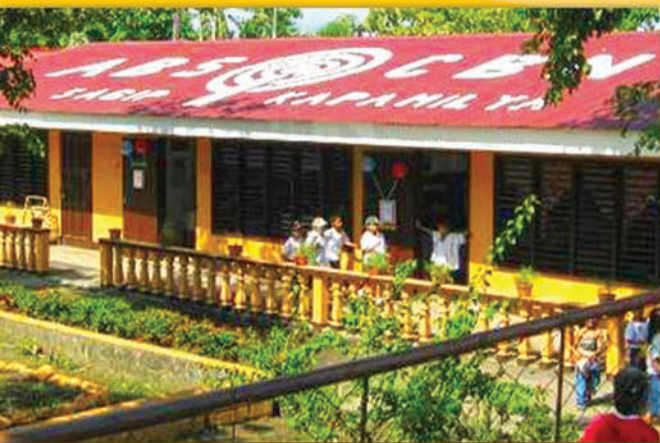
Classroom renovation in Oas North Central School in Albay
